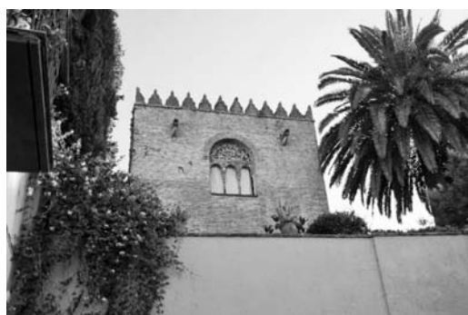
The roof of a walled garden house in Albaicin
